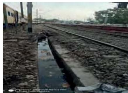
**Figure 4.2: Sewage of Platform No. 05/06 blocked with Ballast at Gaya (ECR).**
