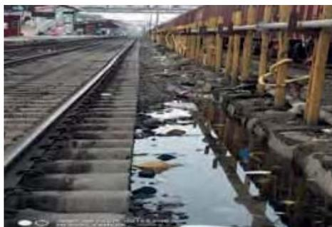
**Figure 4.1: Sewage of Platform No.03/04 blocked with Ballast at Gaya (ECR).**
